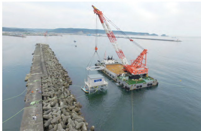
波力発電装置の設置 Construction of wave power generation equipment.
